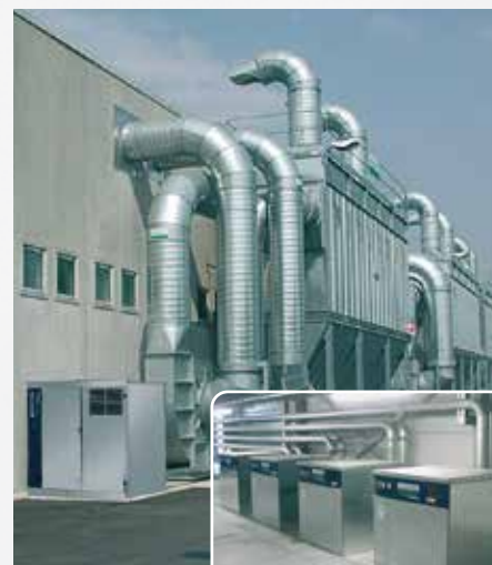
• Industrial: Pneumatic transport of wood chippings ROBOX evolution blower unit
